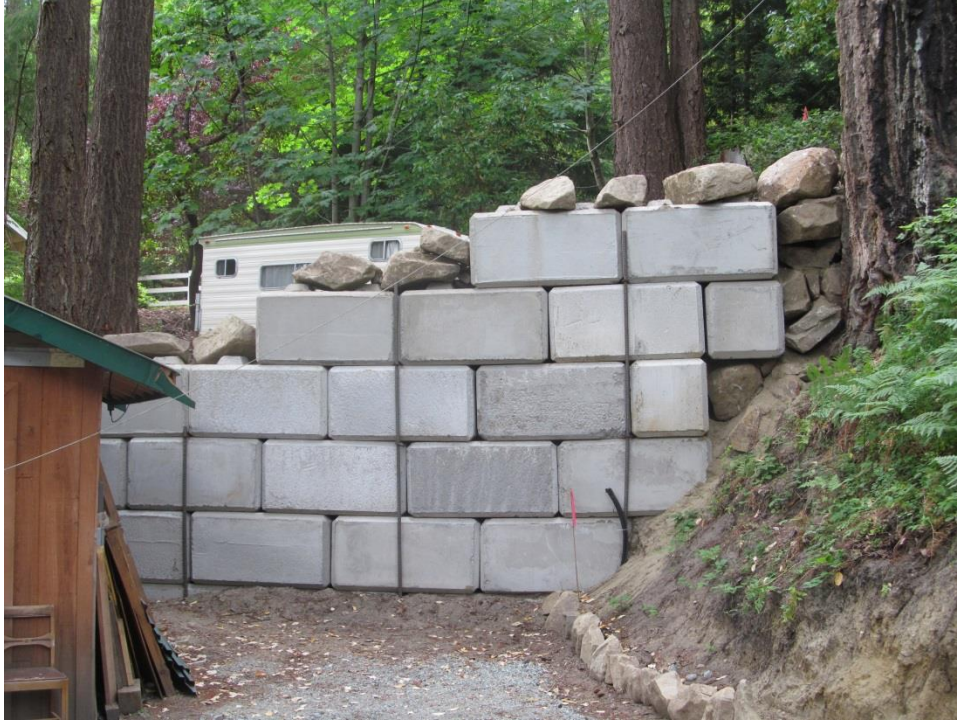
Figure Five: Photo of Retaining Wall (view from adjacent property)
